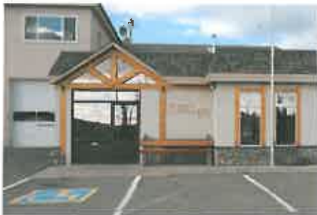
Reflective glass disconnects inside activities from outside activities and parked cars segregate building entrances from the view.
