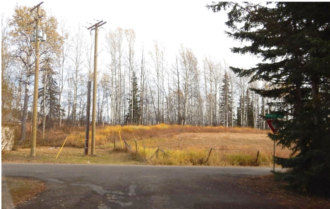
Figure 6: Obscured Yield Sign with Insufficient Sight Distance – Bennett St at Pioneer (Photo 8)
