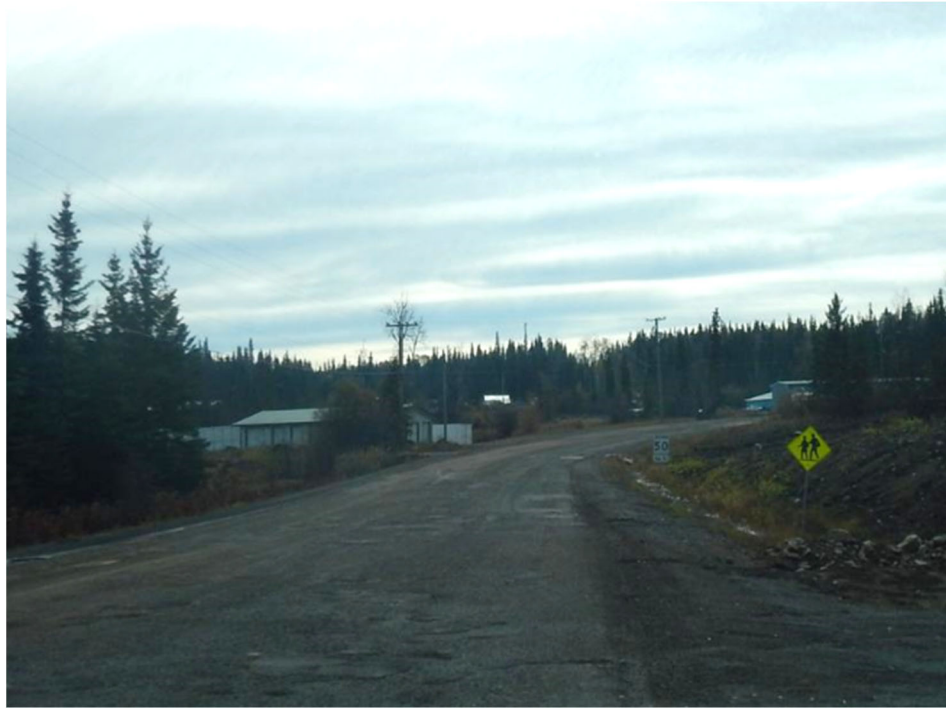
Figure 9: No Crosswalk After Advance Warning Sign – Roumieu Drive (Photo 1)
