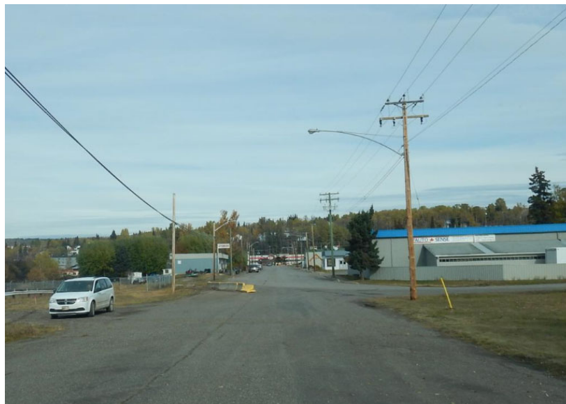
Figure 23: Warrant for New Centreline – Francois Lake Drive at Curve (Photo 20)
