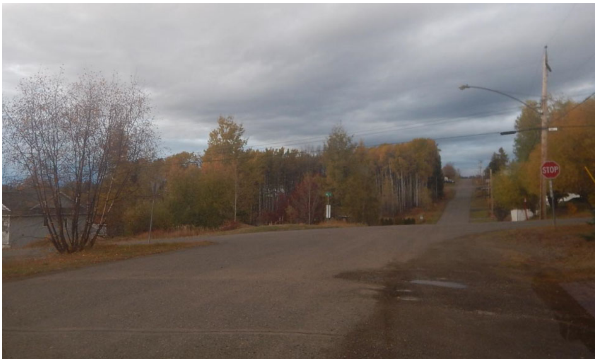
Figure 4: Two Stop and One Yield Sign at Four-Leg Intersection – Carroll Street at Hill (Photo 158)
