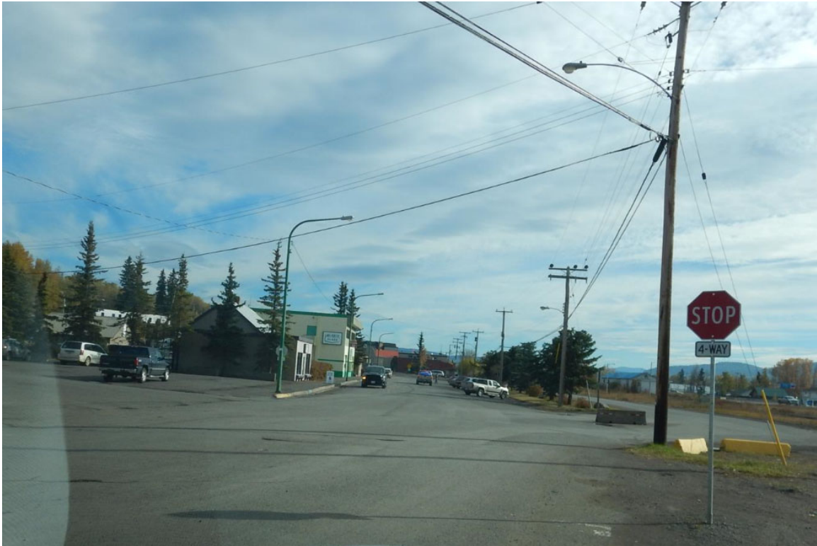
Figure 25: Stop Lines Warranted at Four Way Stop – Government Street at Third (Photo 59)
