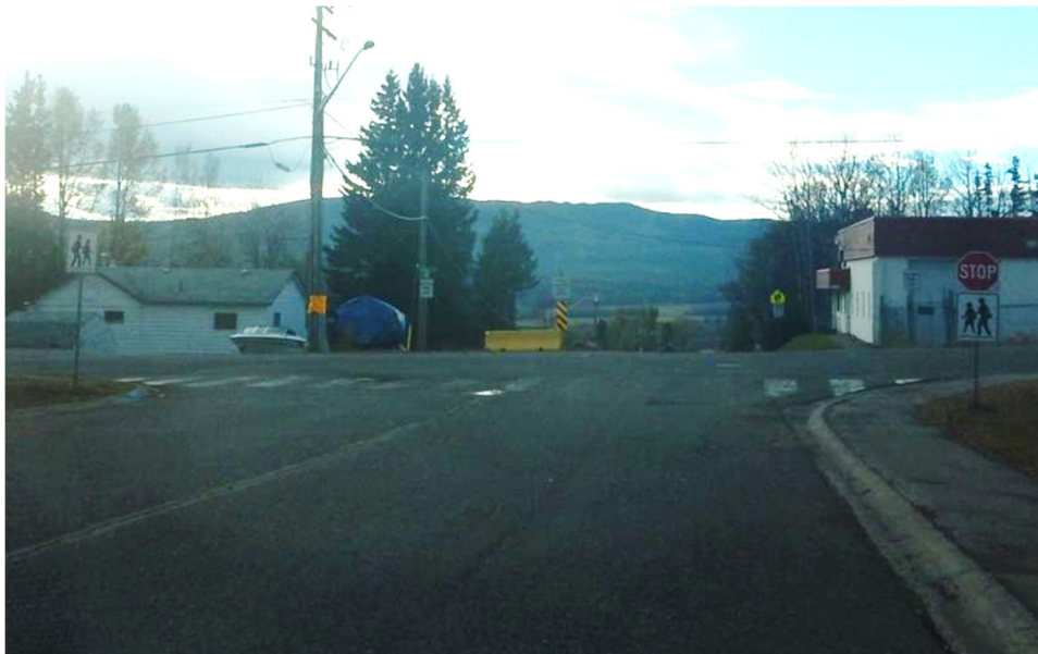
Figure 10: Unwarranted Signs/Markings at Stop Condition – 9 th Ave at Carroll St (Photo 118)
