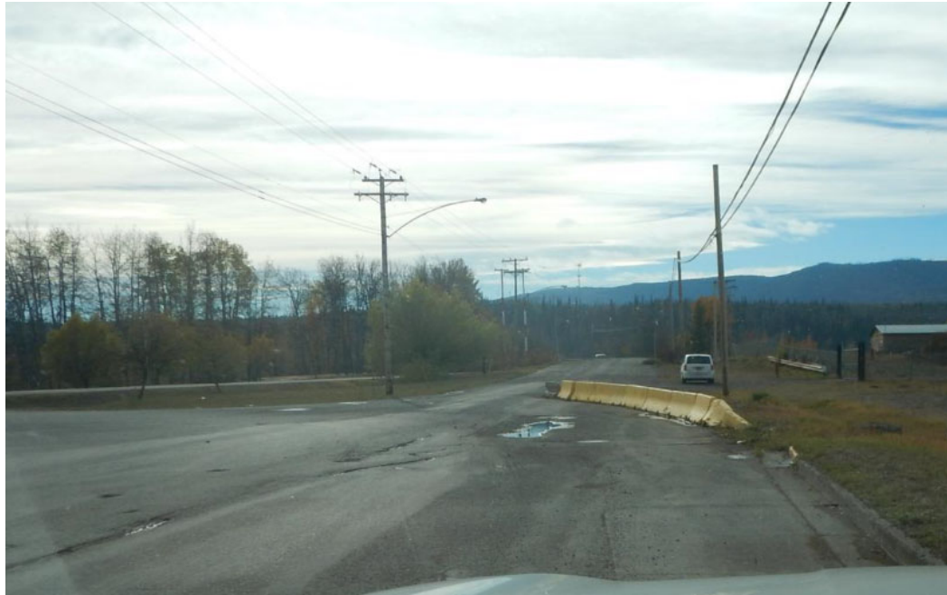
Figure 18: Hydro Poles Need Better Visibility in Road Area – Railway Avenue (Photo 38)
