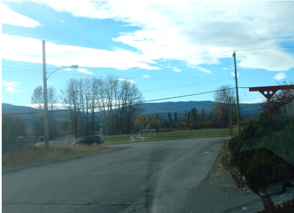
Figure 14: Missing Playground Zone Sign – Fifth Avenue (Photo 65)
