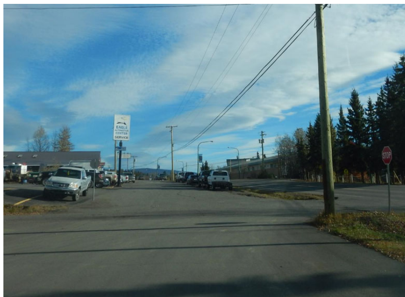
Figure 3: New Stop Signs Warranted at Four Leg Intersection – Highway Frontage Rd (Photo 80)
