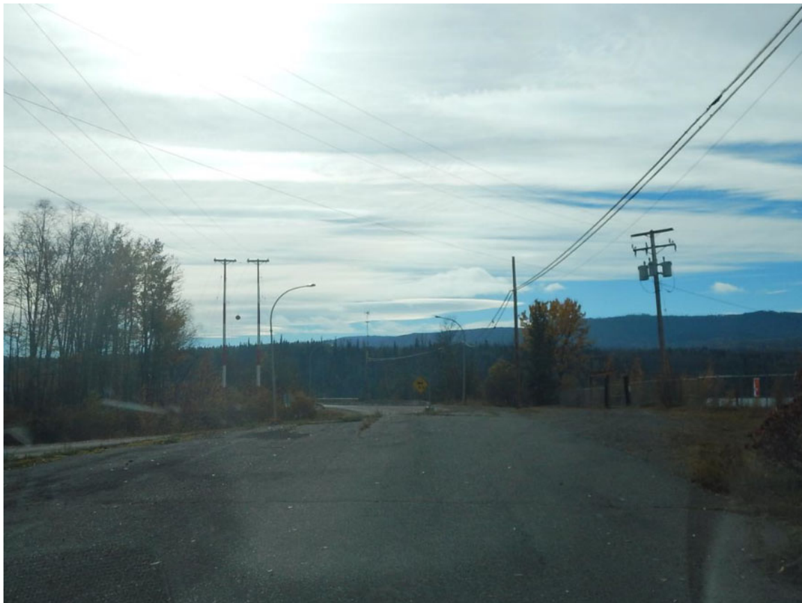
Figure 19: New Checkerboard Warranted – Francois Lake Drive (old section; Photo 19)
